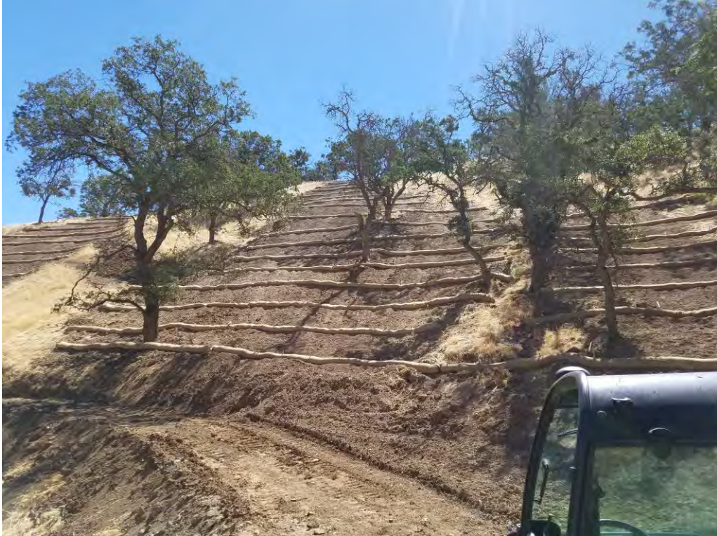
Figure 13: Wattle installation within Black Bear Sub-RMA.
