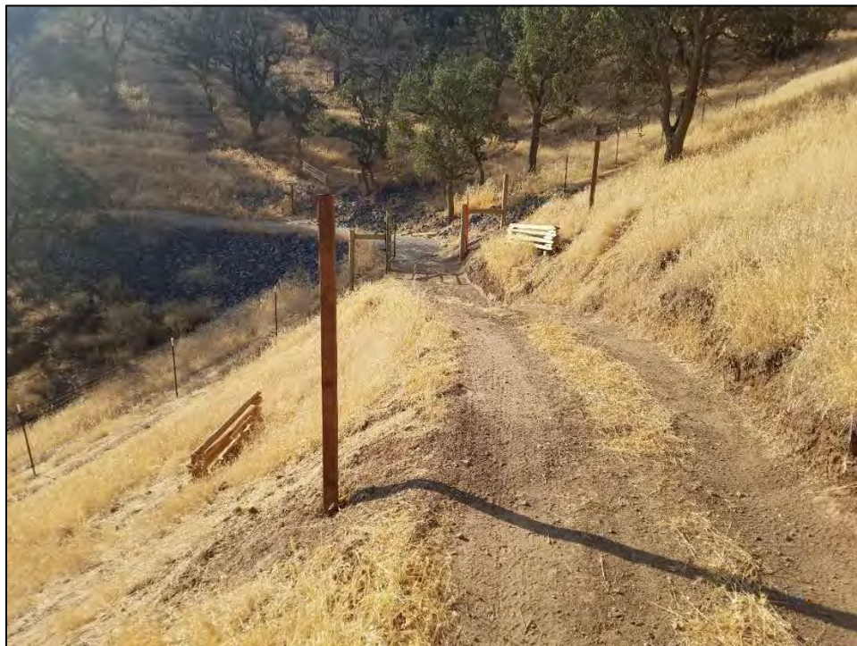
Figure 16: Example of new fencing installed in Black Bear RMA (July 2018)
